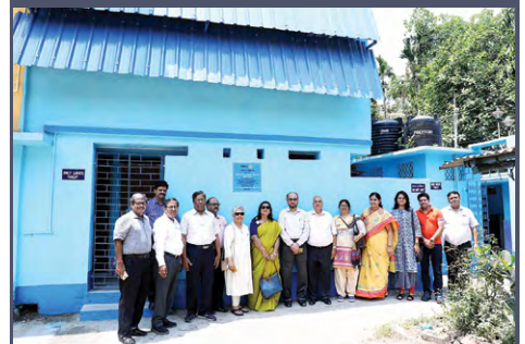
Inauguration of toilet block at Swaika Girls High School in Liluah Howrah, West Bengal by District Governor Shyamashree Sen constructed by Rotary Club of Belur.
