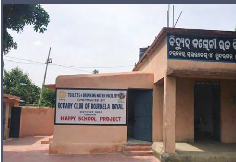
Construction of toilet block and group handwashing station by Rotary Club of Rourkela Royal at Vidyt School Rourkela.
